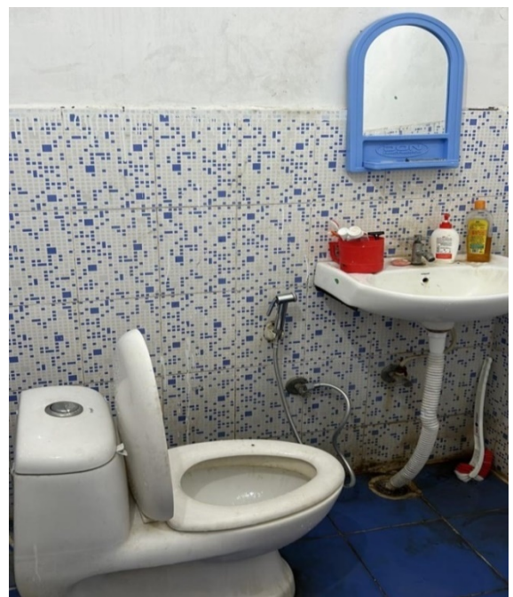
Warden Office Toilet – Boys Hostel
