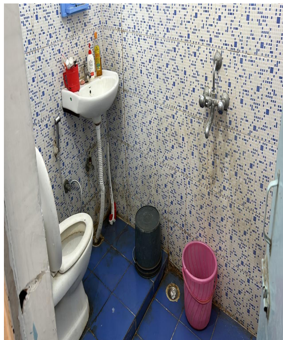
Warden Washroom – Boys Hostel
