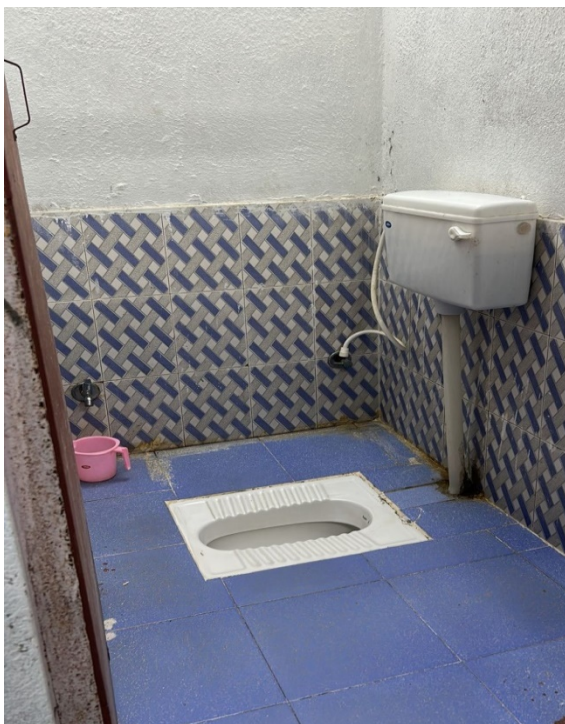
India Toilet – Boys Hostel
