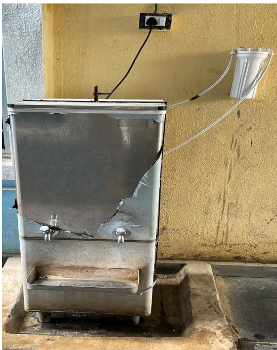
RO Water Cooler – Boys Hostel
