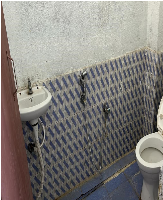
Western Toilet – Boys Hostel
