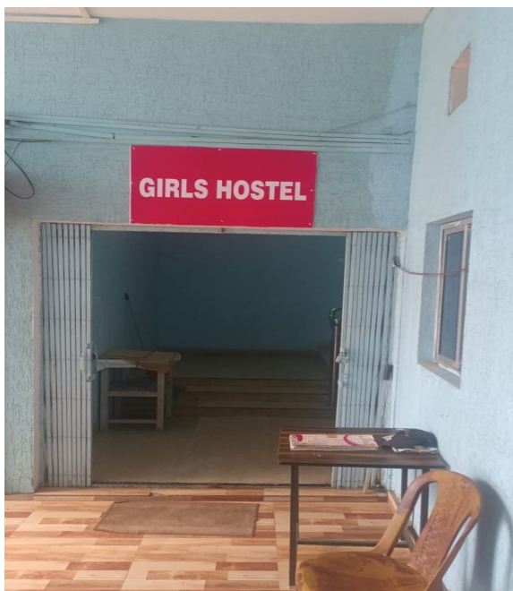
Entrance Gate – Girls Hostel
