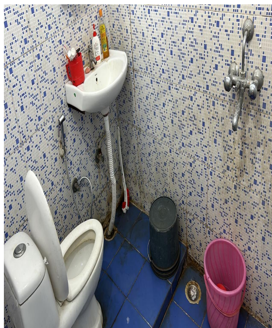
Warden Washroom – Boys Hostel
