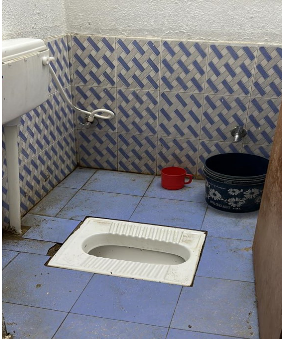
India Toilet – Boys Hostel
