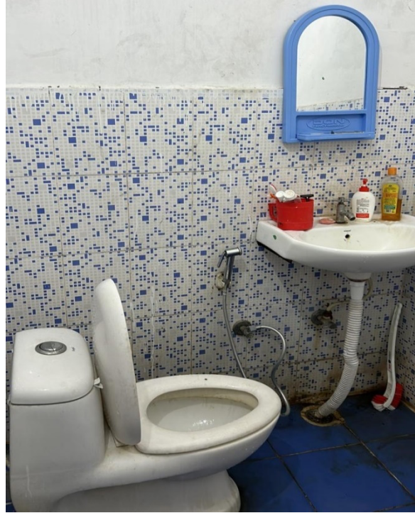
Warden Office Toilet – Boys Hostel
