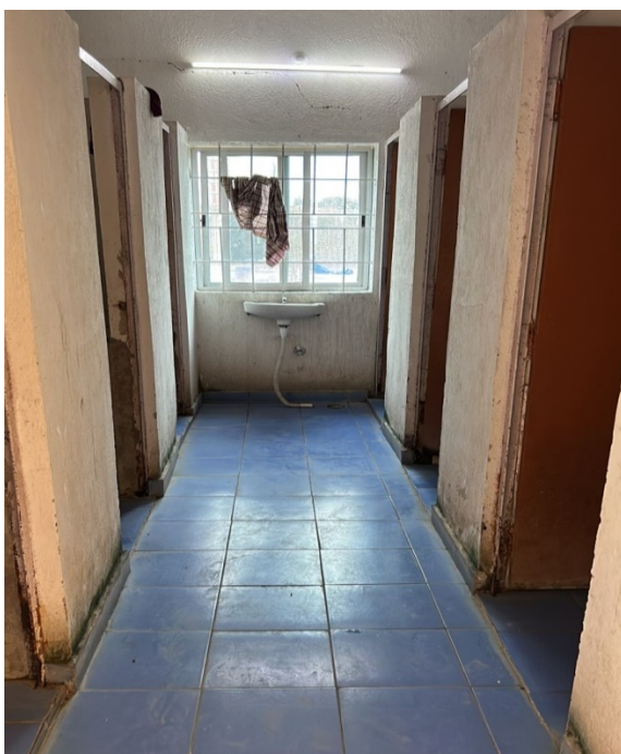
Toilets & Washrooms – Boys Hostel
